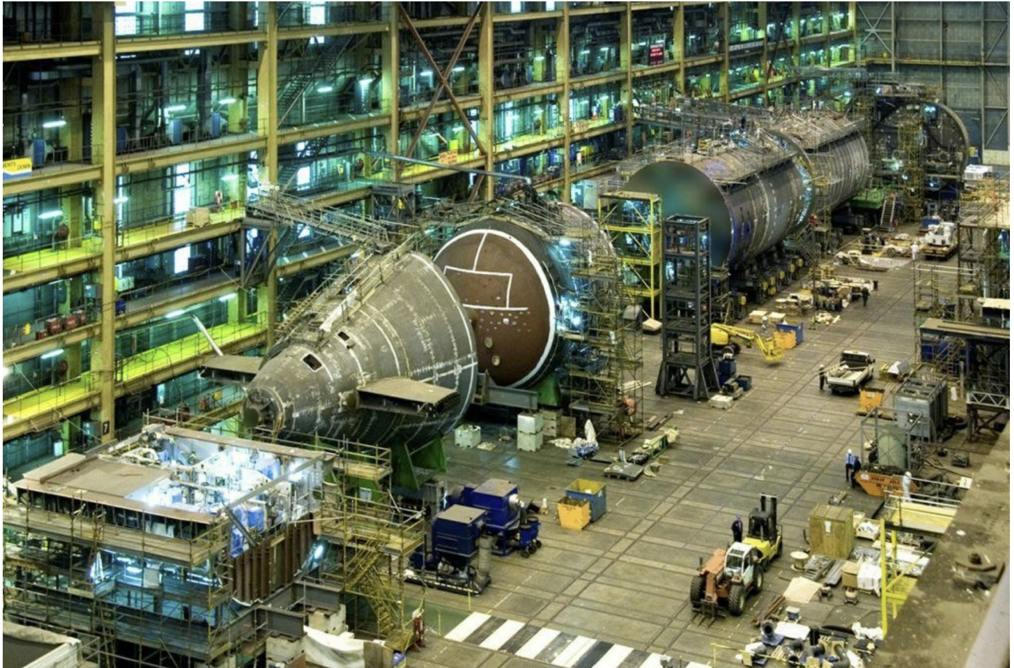
ABOVE: Interior view of the BAE Systems Barrow-in-Furness yard and a nuclear-powered submarine under construction.
